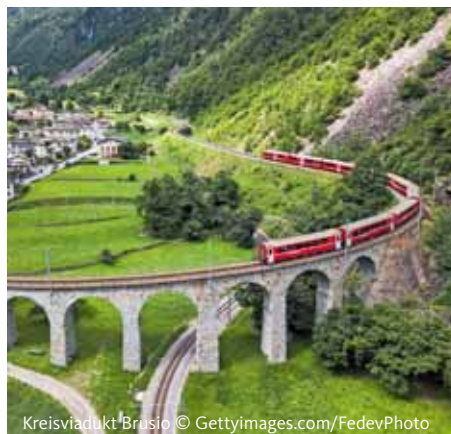
Kreisviadukt Brusio © Gettyimages.com/FedevPhoto
