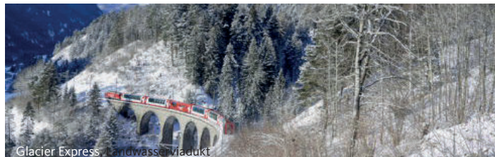
Glacier Express, Sandwasser Viadukt
